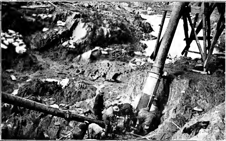
HYDRAULIC ELEVATOR BEING CLEANED JUST BEFORE DISMANTLING
